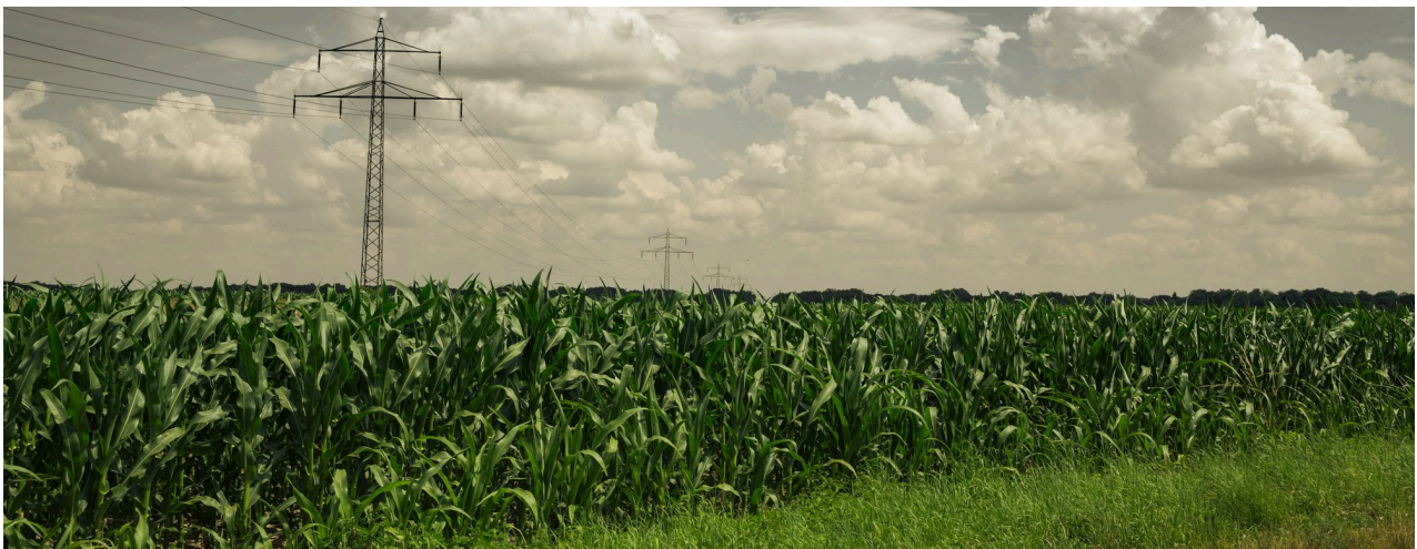
A green maize field with a high-voltage pylon and power lines under grey-white cumulus cloud.
