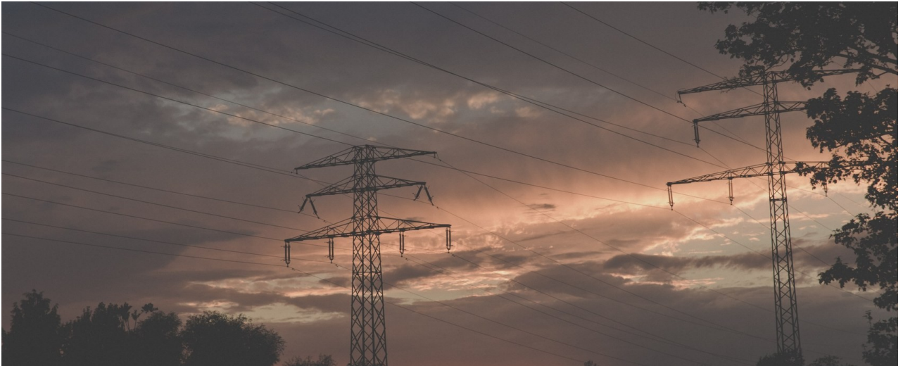
A transmission corridor at dusk with trees standing close to the conductors. Encroachment on a right of way is a change-detection problem long before it becomes an inspection problem.
