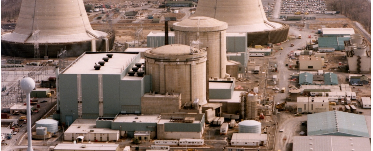
A generating site from the air. One acquisition puts the whole footprint on a single dataset and a single date — buildings, laydown, hardstanding, the vegetation margin and the river beyond it.
