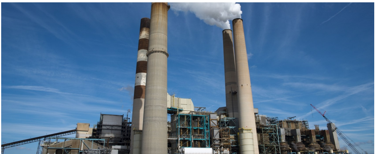
A generating station on the waterfront. Plume, thermal signature, site condition and the receiving water are all surface measurements that one repeat acquisition can carry at once.
